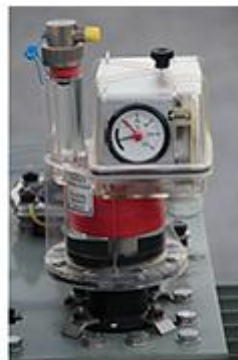
[a] Transformer protection relay (DGPT)
