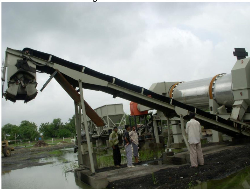
Fig. Load Out Conveyor
